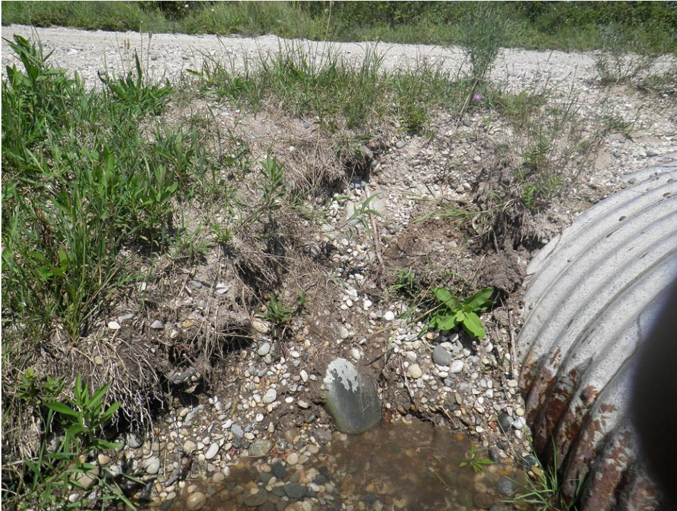
Figure 21: Elliot Creek at Alpena State Road (DG 21)
