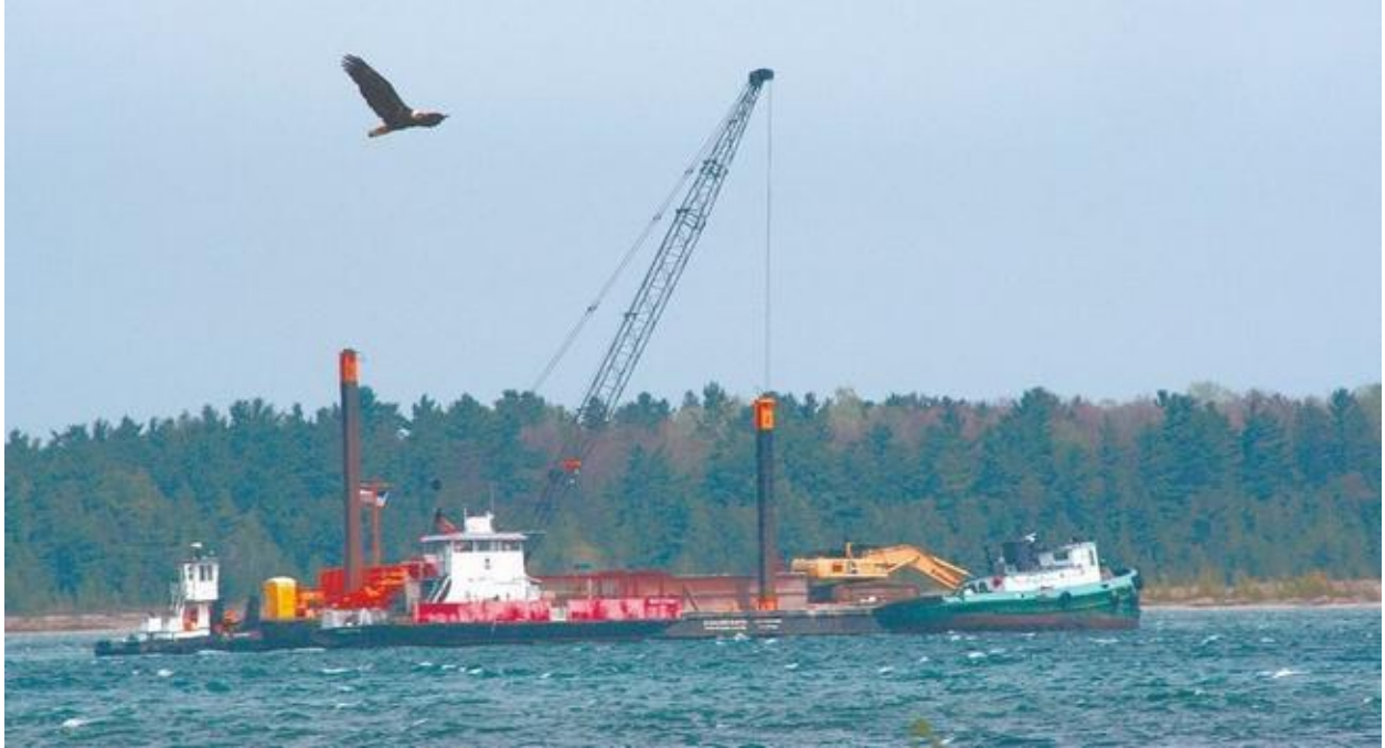
Figure 14: Tugboat Removal (2013) Photo credit: Mike Fornes/Cheboygan Tribune
