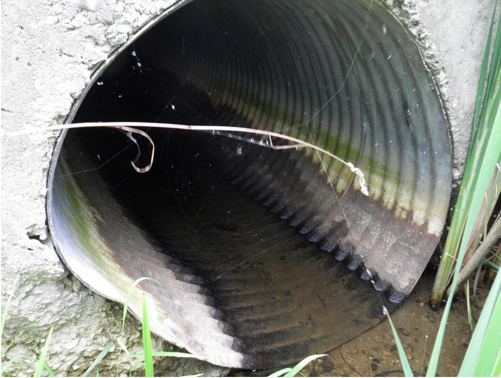
Figure 20: Butler Ditch culvert under Butler Rd. (DG 01)
