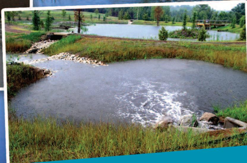
Although less biodiverse than natural wetlands, they can provide adaptation functions by providing habitat, corridors, shade, microclimate benefits during hot spells, and greater aesthetic values than traditional stormwater ponds. They can provide nutrient uptake and groundwater recharge. Stormwater wetlands are much less likely to become full of algae and stagnant water, and are designed to function more like natural systems than traditional stormwater basins.
