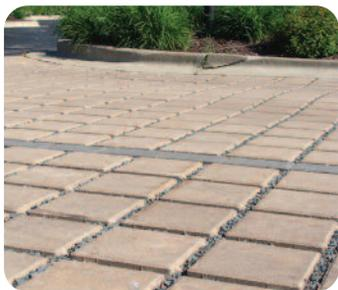
**Permeable pavers** are comprised of interlocking concrete bricks, separated by joints or gaps, filled with small stones or sand, which are laid over a bed of aggregate stones. Water is able to infiltrate through the joints in the paver and is stored in void space in the stone bed underneath the paver surface, where it is then filtered back into the soil.
