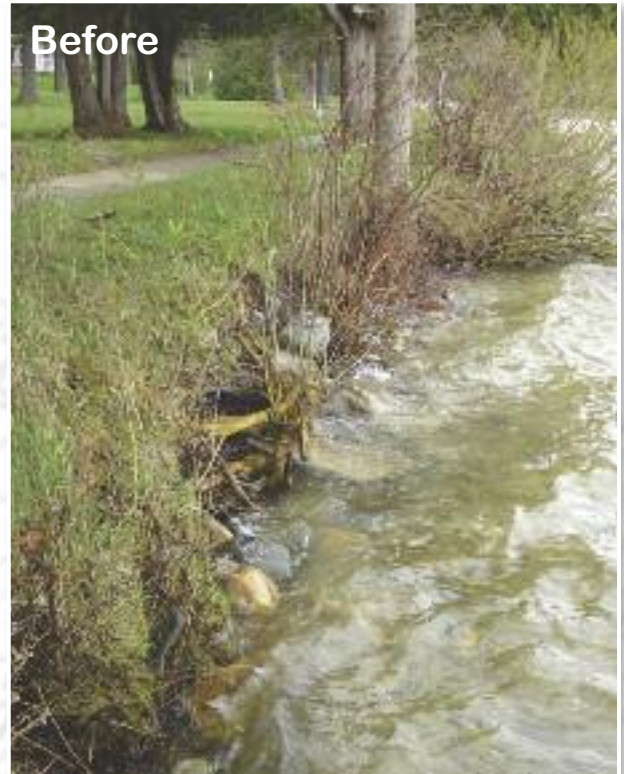
Exposed roots and undercutting along the Columbus Beach Club shoreline as indicators of moderate to severe erosion.
