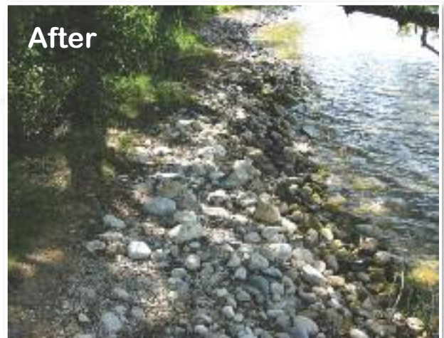
Nearly a year after installing a bioengineering project, the Columbus Beach Club shoreline remains stable and protected.
