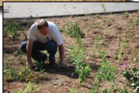
Rain garden installation at the Charlevoix Library.
